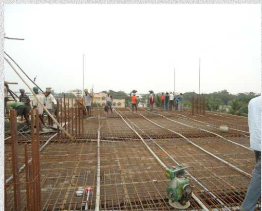
Slab constructed with the service of Nirmaan Sanjeevani at Tanuku
